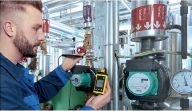
To operate in an energy-saving, comfortable and fail-safe manner, perfect adjustment, and function are crucial for heating systems. During commissioning and maintenance, temperature measurements, e.g. on supply/return temperatures, show whether the optimum operating condition is ensured. After hydraulic balancing sound heat distribution can be checked quickly and reliably with the G 1202.
